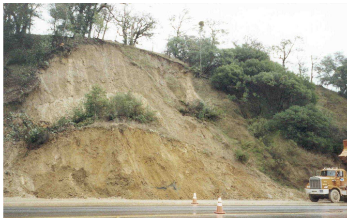
Figure 1.1: Slope failure initiated by an extreme rainfall event ( www.dot.ca.gov/hq/esc/geotech/photos/north/north.htm ).
