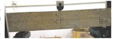
(a) failure pattern of plain concrete beam
